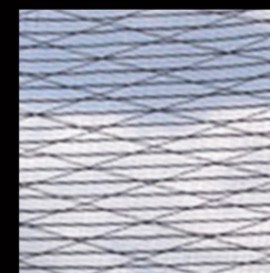
ETFE REINFORCEMENT: DYNEEMA FIBER
